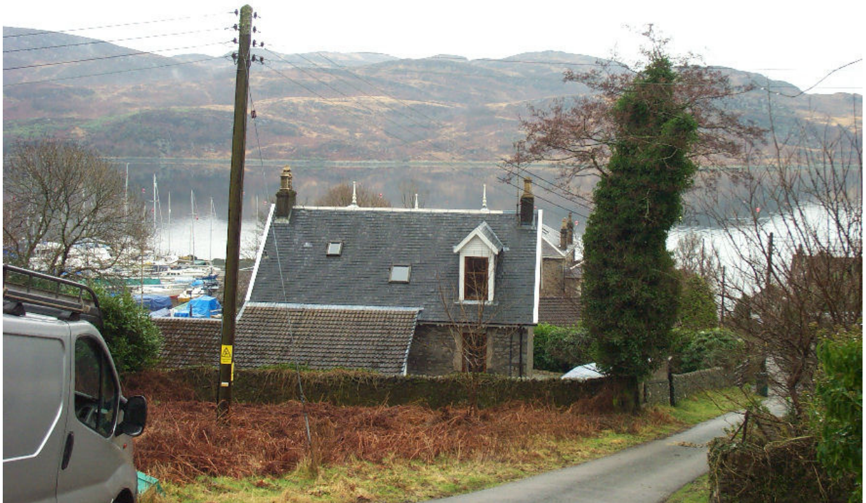
Photo_08 Aldersyde rear view.
