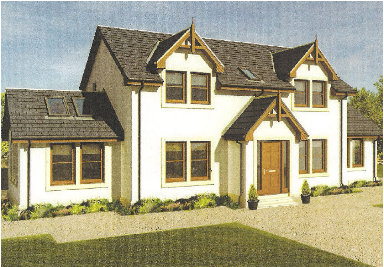
Orange House (Scotframe Timber Engineering).
